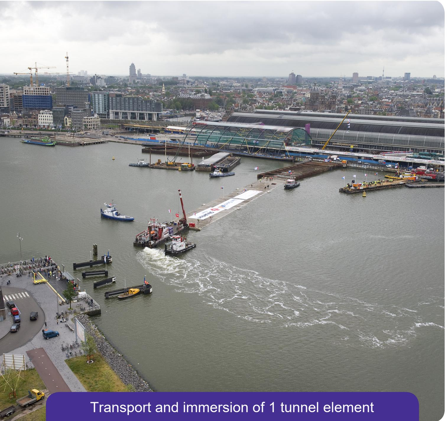
Transport and immersion of 1 tunnel element
